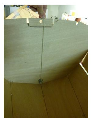
Push the moulds provisionally in place between the planks in their installation position and then check whether they are plumb.
