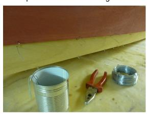
... and assemble them loosely together. The two planks are fitted exactly **edge to edge**.
