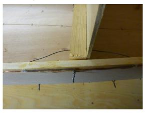
This is what it should look like: The plank 2 is fixed over the entire length of plank 1, two frames are installed:
